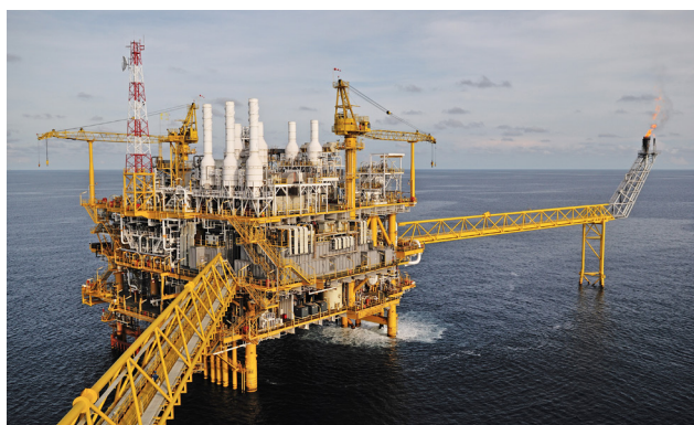
Figure 4: The off-shore platforms for oil production are linked to sub-sea CANopen networks comprising redundant controllers, different sensors, valves, and other equipment (Source: Adobe Stock)
