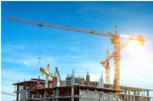
Figure 4: CANopen networks are used in vehicle-mounted lifting equipment. Wika, for example, uses CANopen Safety for overload protection purposes in container, gantry, lattice boom, telescopic, and other cranes. (Source: Adobe Stock)
